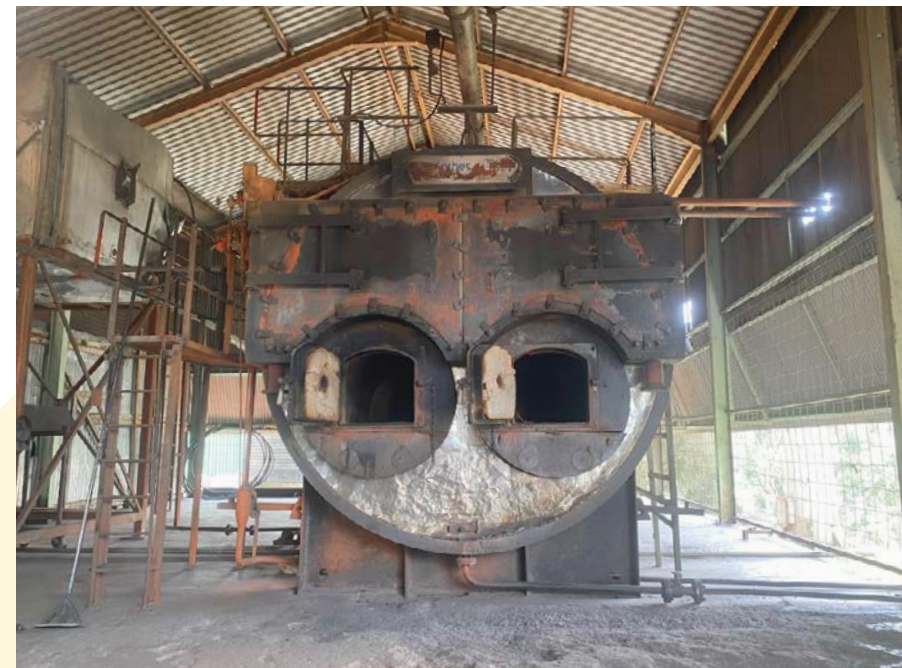
FIGURE 6. Wood fired boiler furnace at a tea processing facility
