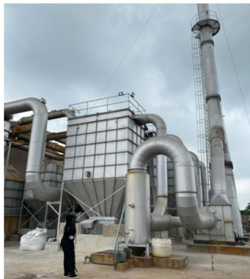
Off-gas treatment system with cooling towers, baghouse, scrubber and stack
