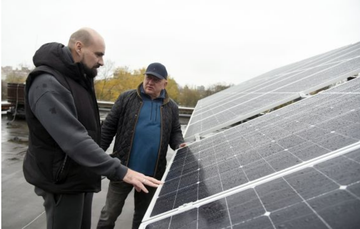
Installed solar panels at children's hospital in Ukraine © GIZ
