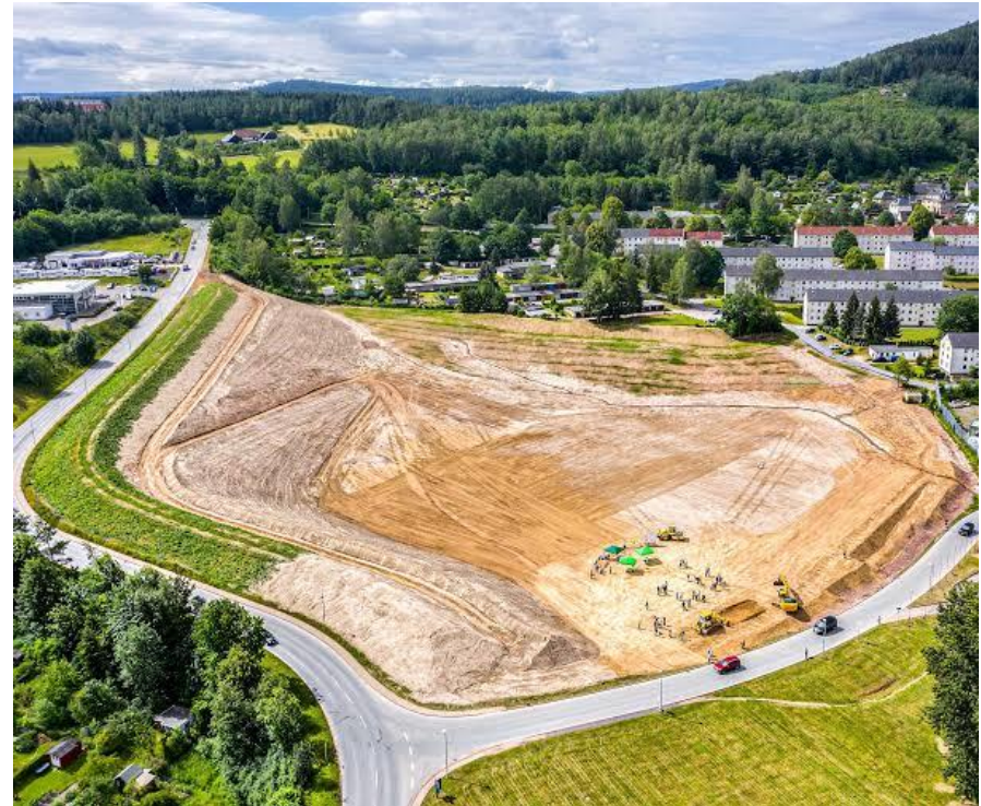
Part E Chapter 4 Figure 9. Example of a rehabilitated landfill.
