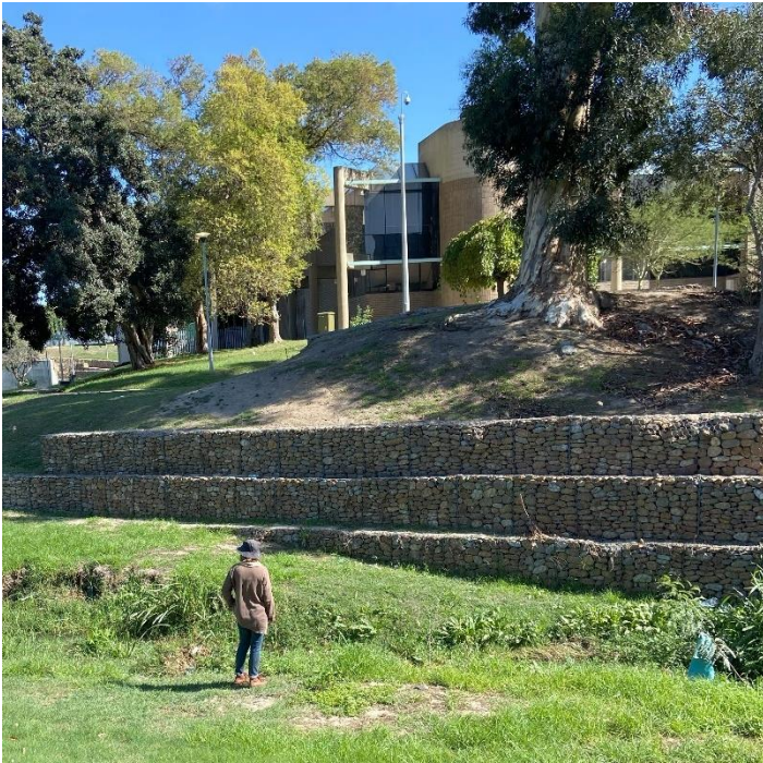
Part E Chapter 4 Figure 13. Example of terraces gabion walls.
