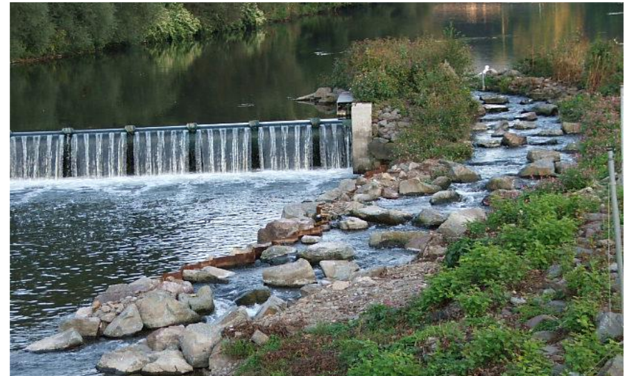
Part E Chapter 3 Figure 4. Examples of constructed natural bypasses for fish movement in Germany (above) and Finland (below) (from Bok et al., 2007).
