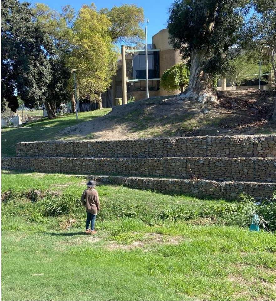
Part E Chapter 3 Figure 6. Terraced gabions
