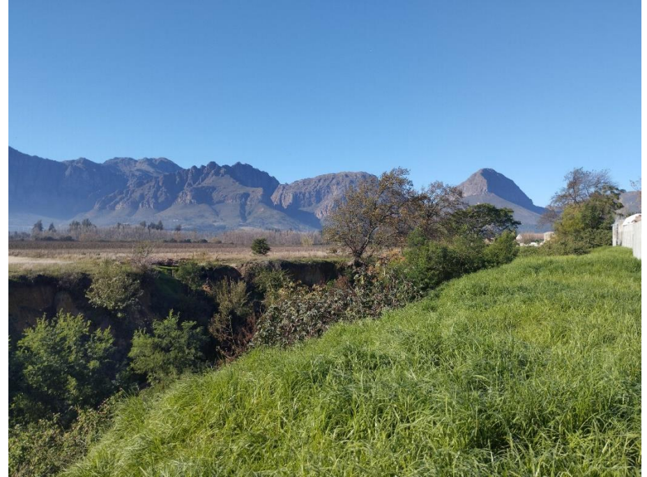
Part E Chapter 3 Image 2. This section of the river is deeply incised with eroded embankments.
