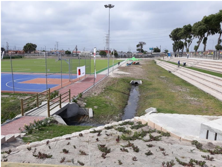
Part D Chapter 3 Figure 5. Sports field with swale and seating (Source: Plan prepared by Design Space Africa and provided by City of Cape Town Catchment Stormwater and River Management Branch).
