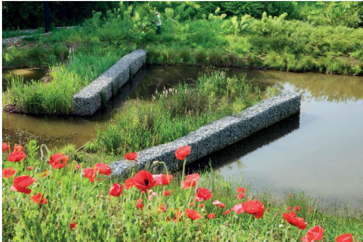
Part D Chapter 3 Figure 4. Gabion structures in a treatment wetland (Source: https://www.hargreaves.com/work/chattanooga-renaissance-park/ ).
