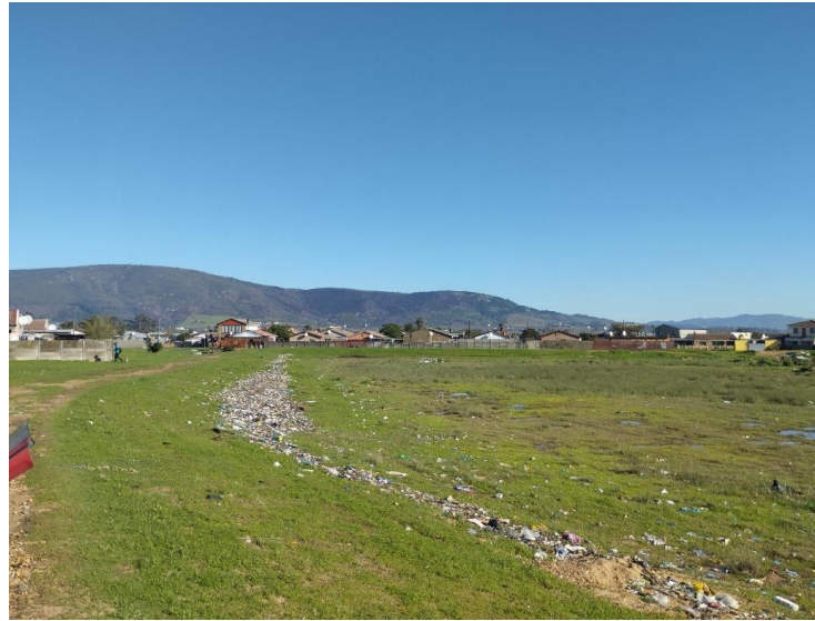
Part D Chapter 3 Image 1. This shows visible solid waste pollution within the detention pond.
