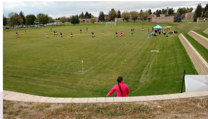
Part D Chapter 3 Figure 8. Precedent image of a multi-use sports field stormwater retention pond ( https://tdengineering.com/project/upgf-multiuse-athletic-field-intermittent-storm-water-detention-pond/ )
