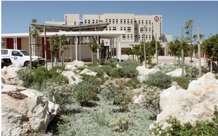
Part D Chapter 3 Figure 11. Planted swale at Mitchells Plain District Hospital
