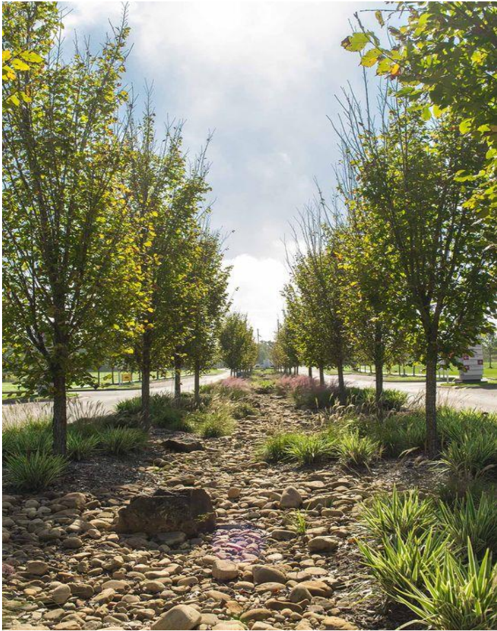
Part D Chapter 3 Figure 12. Planted swale
