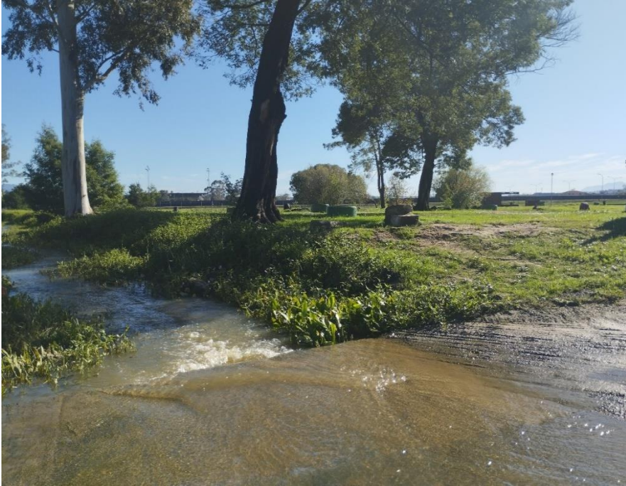
Part D Chapter 4 Image 1. This shows how the Boontjies River overtops the road that fragments the river after heavy rain.
