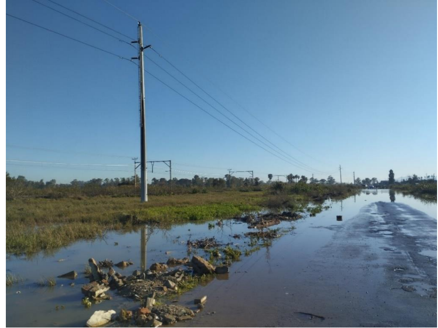
Part C Chapter 4 Image 2. After heavy rains, Drommedaris Street was flooded - reduced accessibility between the informal settlement and the industrial area.
