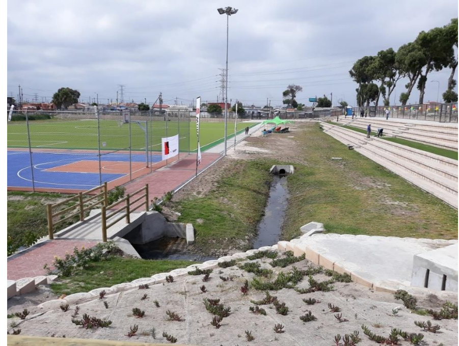
Part C Chapter 3 Figure 15. iThemba Labantu Centre Soccer post-construction (Source: Plan prepared by Design Space Africa and provided by City of Cape Town Catchment Stormwater and River Management Branch)
