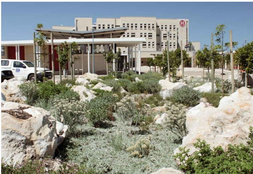
Part C Chapter 3 Figure 16. Planted swale at Mitchells Plain District Hospital
