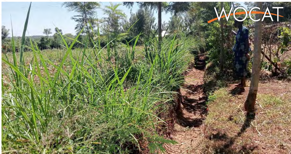
A retention ditch dug to collect surface runoff (William Akwanyi)
