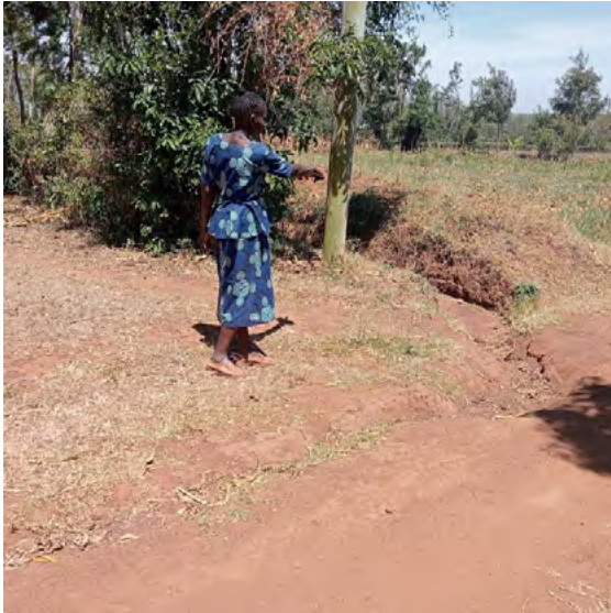
Surface runoff collector at the road (William Akwany)
