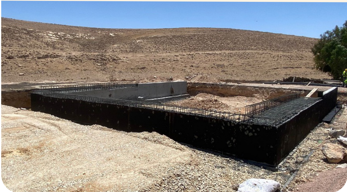
Retaining wall construction
