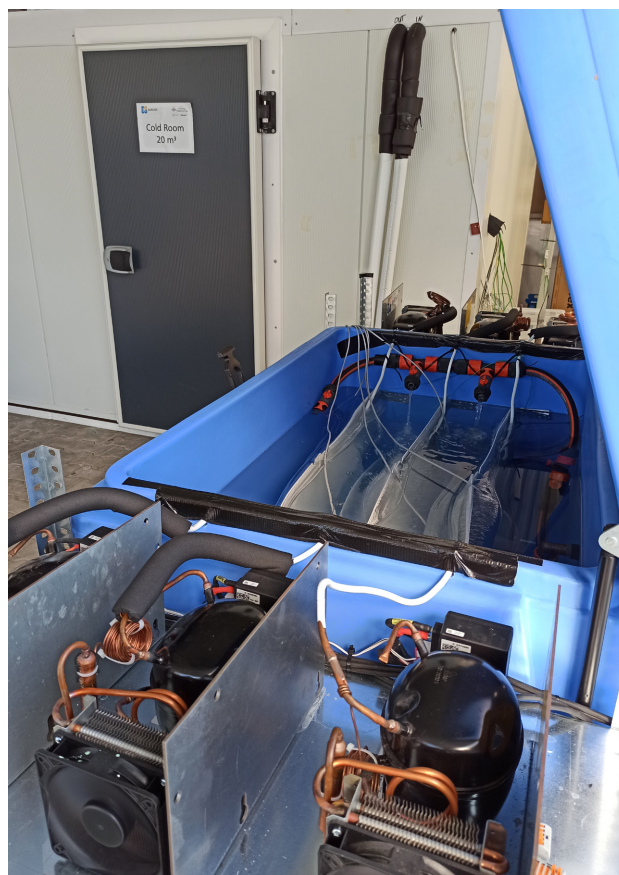
Picture 3: R600a compressors and ice storage solar cold room, © SelfChill Innovation Center, Germany
