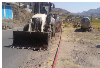
Rehabilitation and extension of Drinking Water Supply Network in Ibb city.
