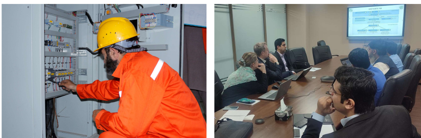
Pg. 1, Left: Local people trained in Chitral overseeing the operation of a small hydro-power plant.
