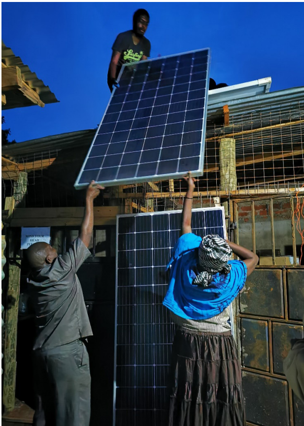
Picture 8. Solar panel is installed with local resources in Kenya.
