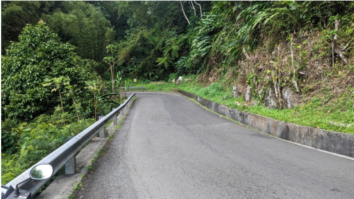
Figure 14: Picture of road type A
