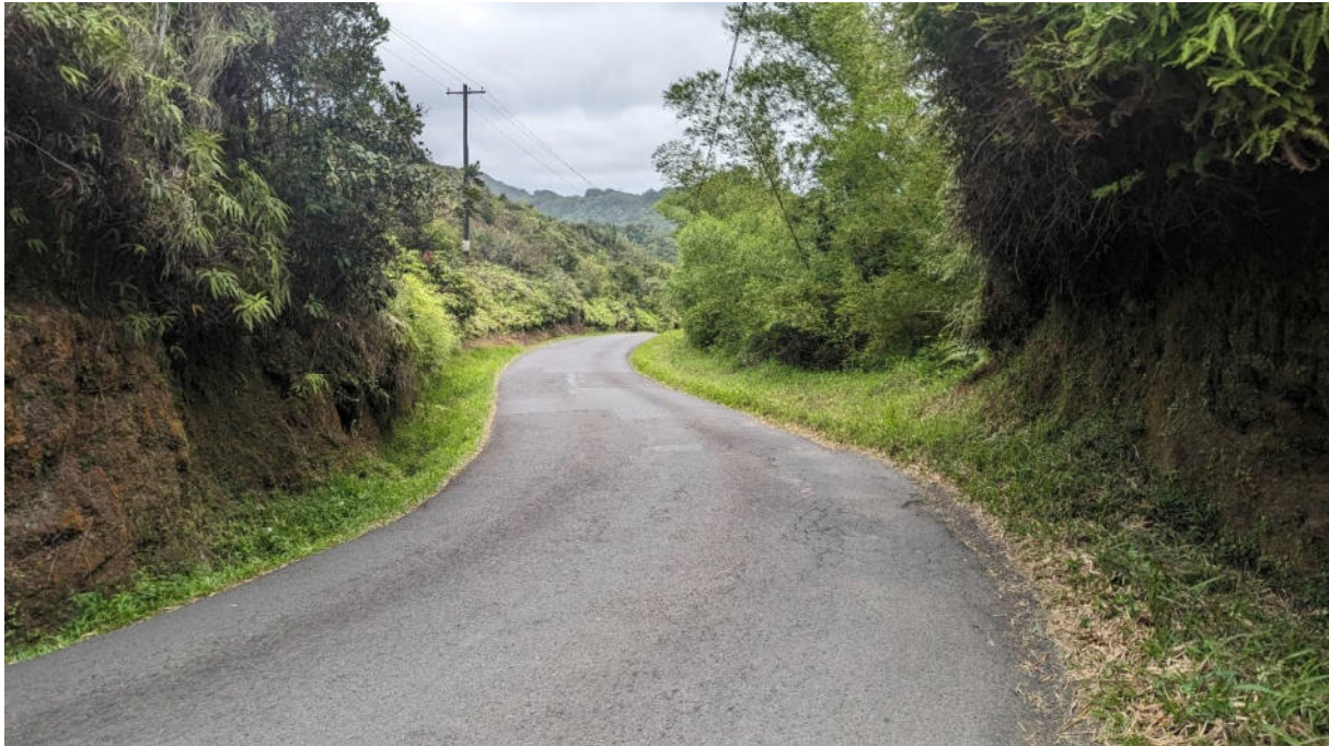
Figure 16 : Picture of road type B
