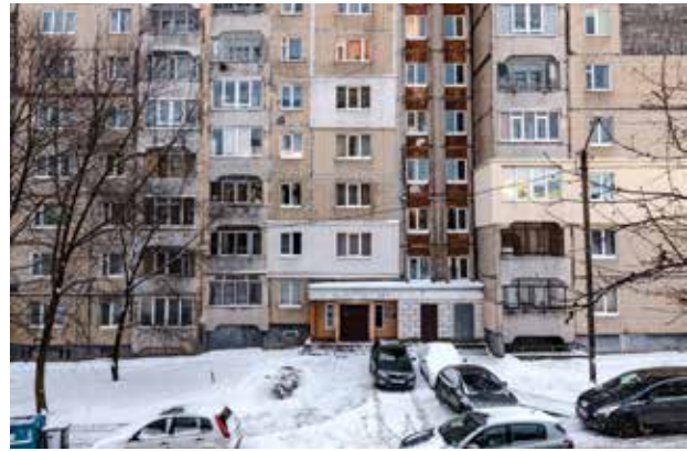
Before refurbishment: The façade of a residential building in Lviv, Sychiv district, which is set to become an energy-efficient neighbourhood. A lot of energy is lost due to inadequate insulation.
