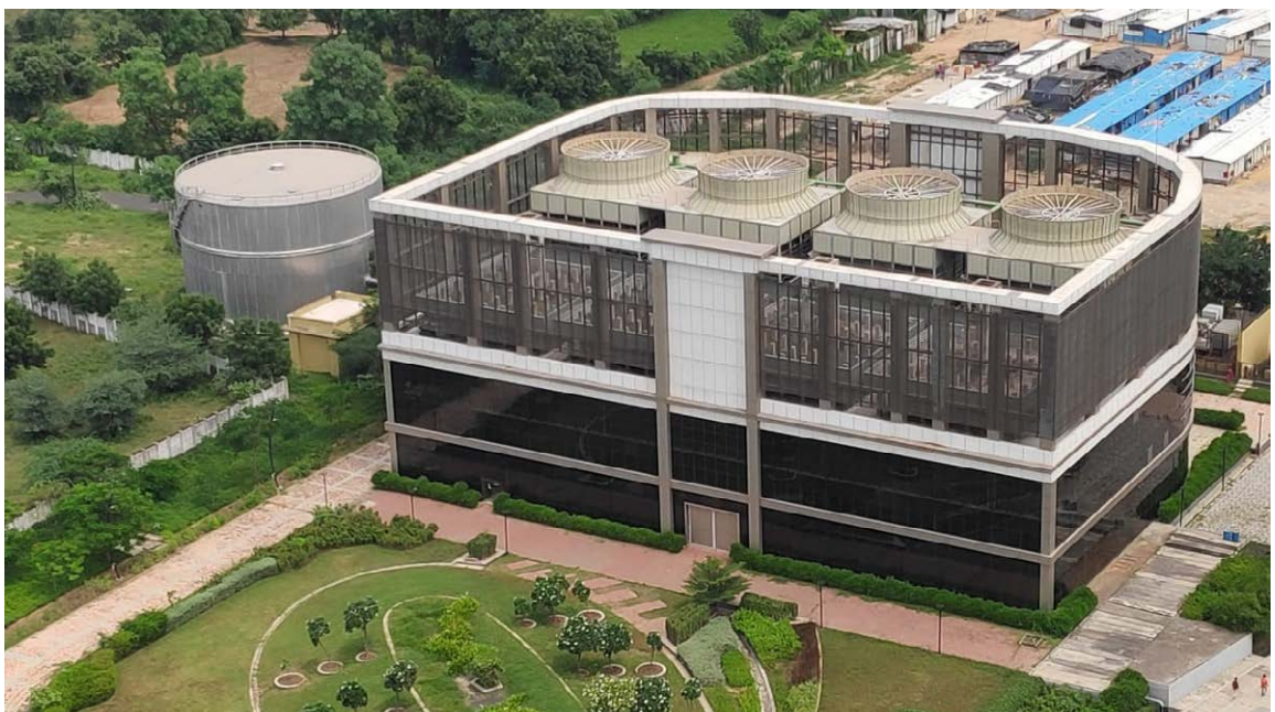
Figure 20: GIFT City DCS: View of DC Plant and TES Tank
