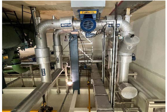
Figure 24: GIFT City DCS: View of Pump Installation
