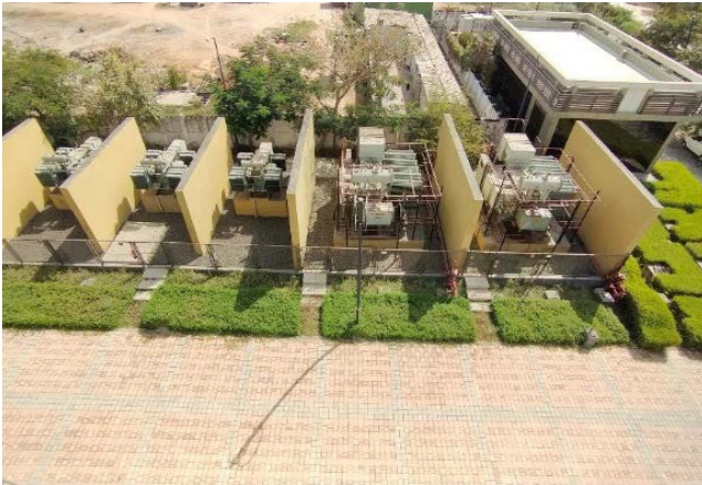
Figure 23: GIFT City DCS: View of Transformer Yard
